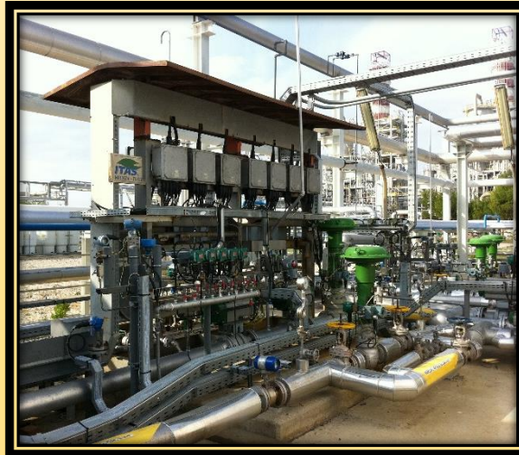
NEW CONTROL SYSTEM
