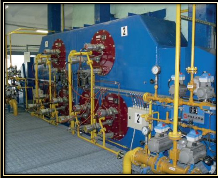
UTILITY BOILER BURNERS
